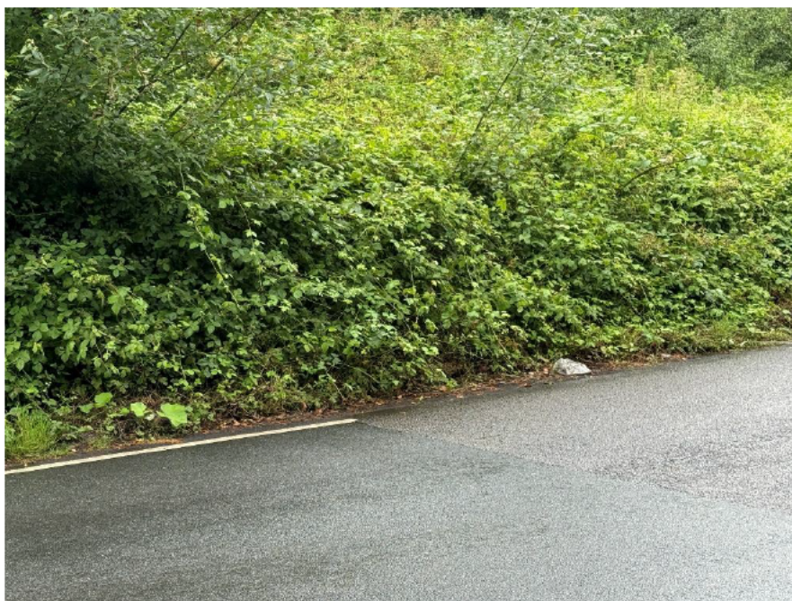
Drainage for the site and for Church Road is within this verge to the site which is no longer being maintained. 3 gulleys are located in view of this image, all covered.
