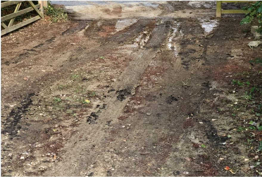
Resulting damage to driveway from clay & silt deposits due to flooding.
