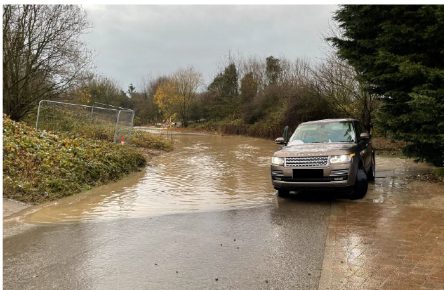
Example of frequent flooding on Church Road during construction due to poor maintenance of existing drainage.
