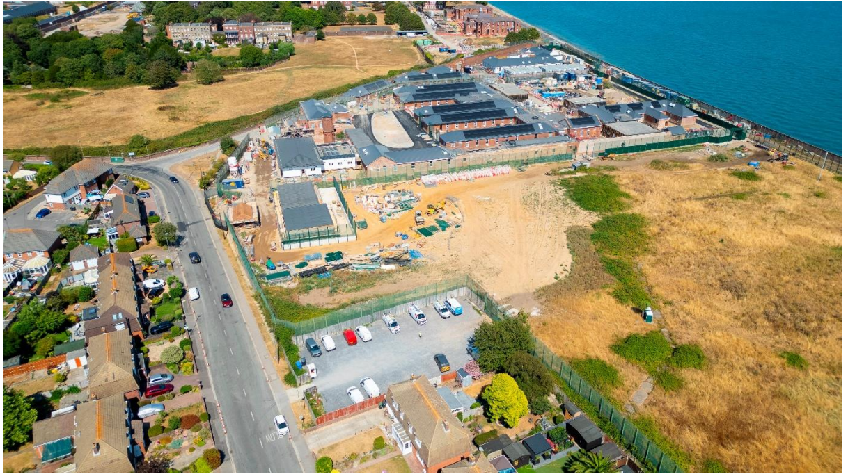
Photo 4 taken July 2026 showing the extent of the energy centre development and how widespread the site works are for such a relatively small section of the development.
