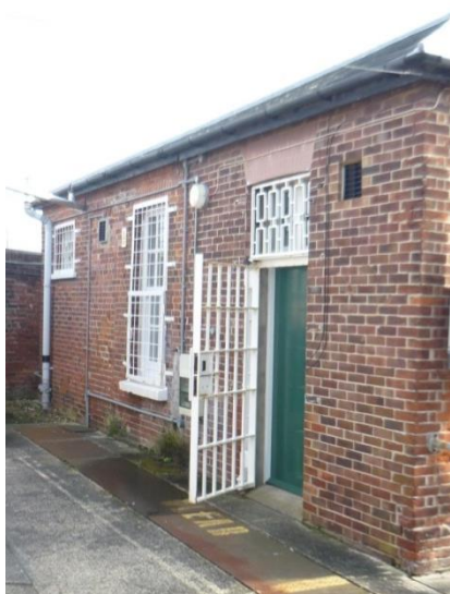
The Guardhouse (northern elevation)
