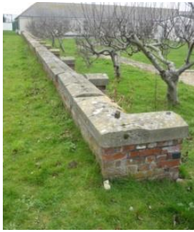
Plinth Wall for railing
