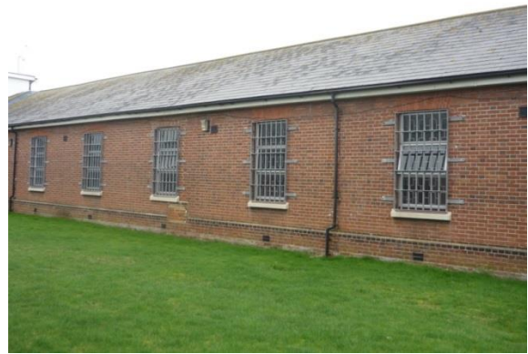
The barrack ranges showing the southern most slightly projecting bay and precise rhythm of elongated openings with rubbed brick lintels and stone cills. Under floor ventilation can be seen within the plinth.
