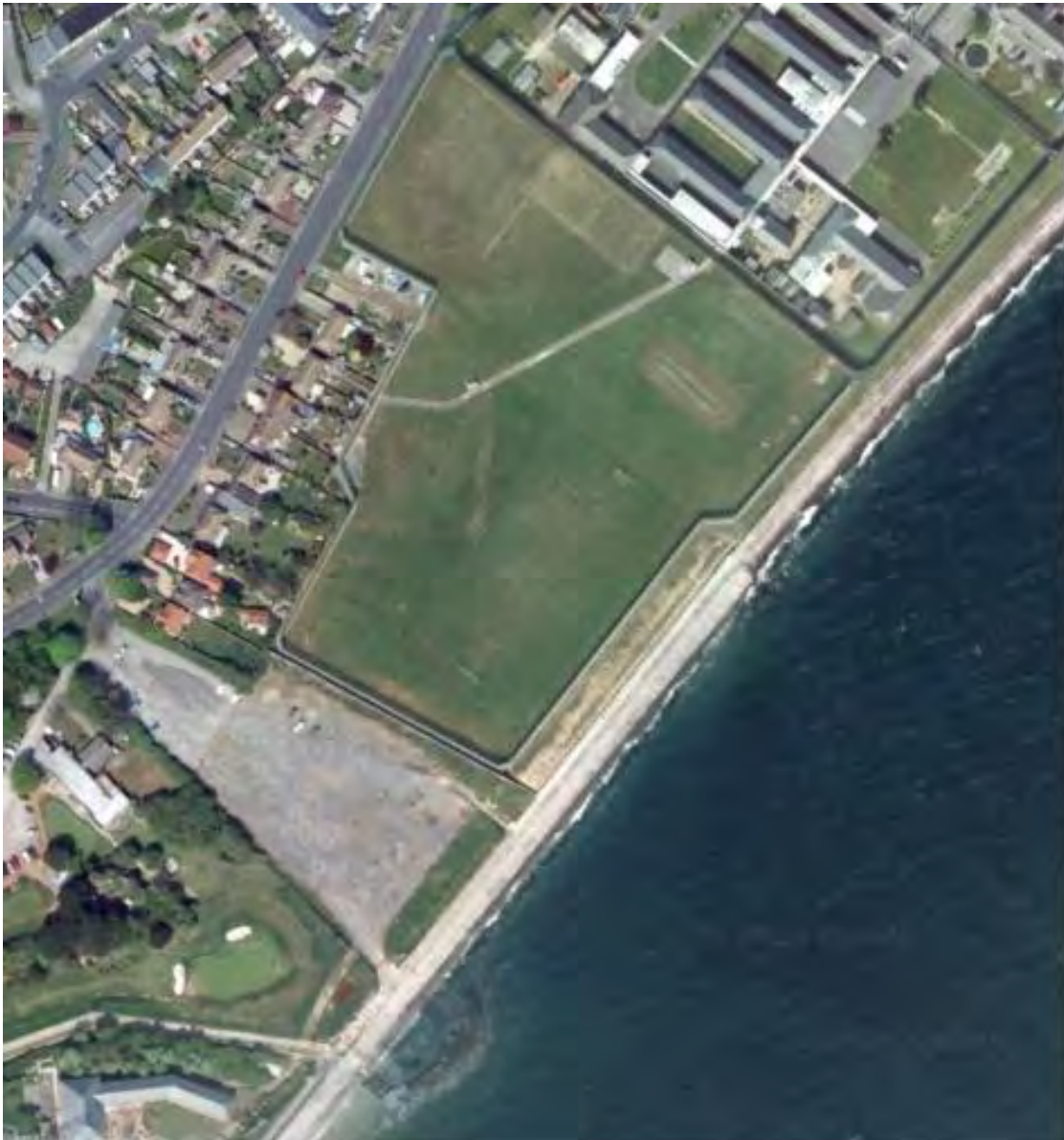
Figure 6.1 – 2007 photograph of Haslar Sea Wall Car Park (source: GoogleEarth).
