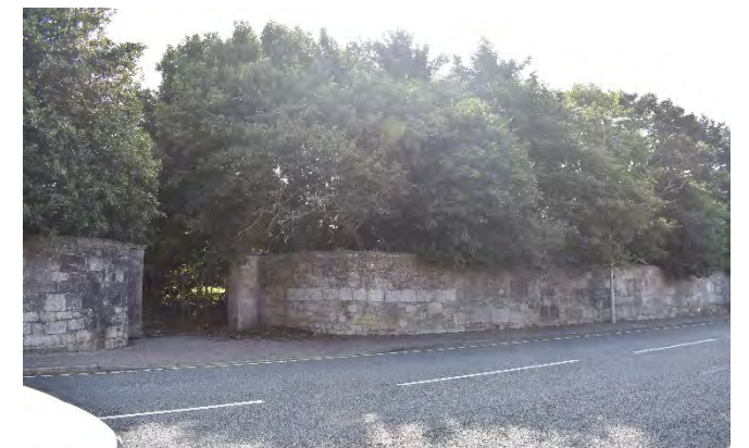
6.22 Historic wall boundary to former Ashburton House
