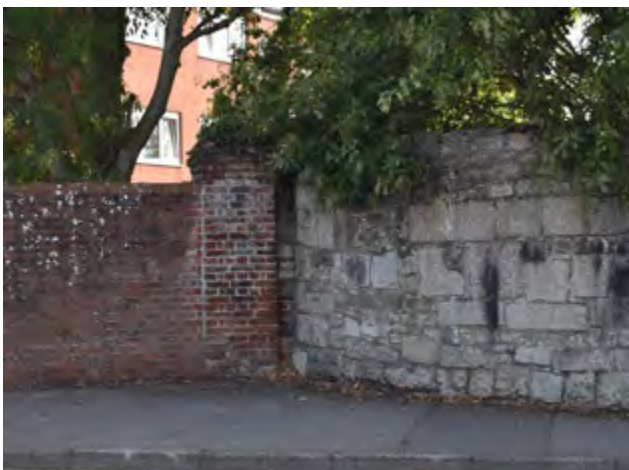
4.19 Combination of stone and brick walls
