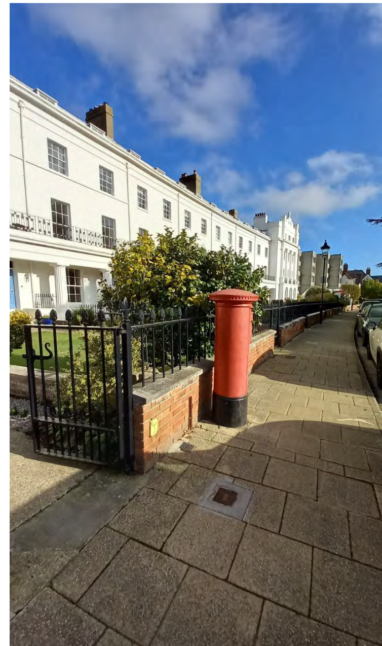
6.13 Regency architecture of The Crescent
