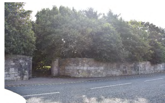
6.22 Historic wall boundary to former Ashburton House
