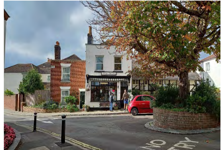
4.5 Stuccoed C19th facades may mask earlier buildings
