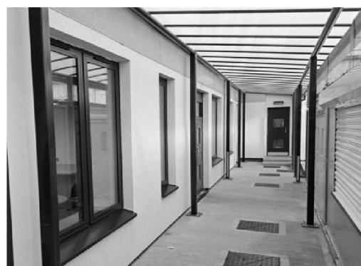
Fig. 12 – Existing Main Building
