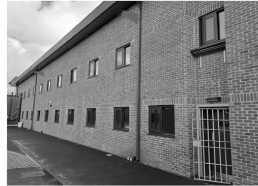
Fig. 8 – Existing Accommodation Block
