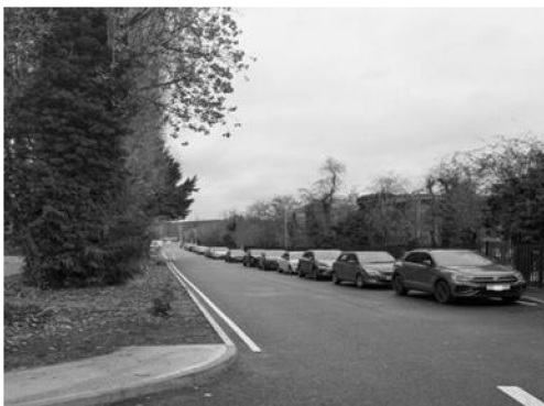
Fig. 3 – Entrance Road leading to Langford Road
