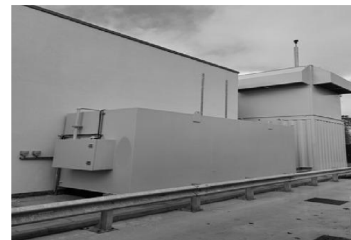
Fig. 10 – Existing Plant Space, Chimney etc.
