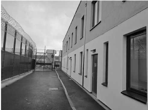
Fig. 7 – Existing Main Building
