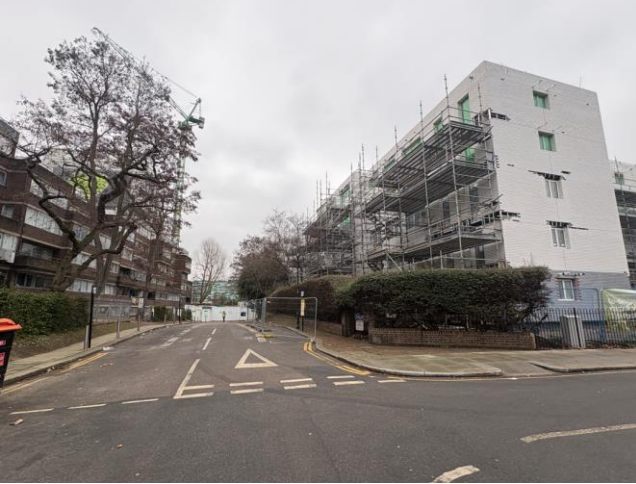
Figure 4-8 – Approach to Site on Treadgold Street
